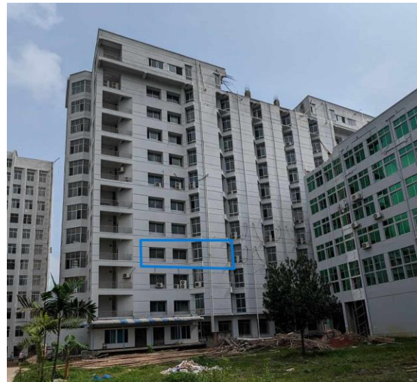
Fig. 05: South facade of the study building
