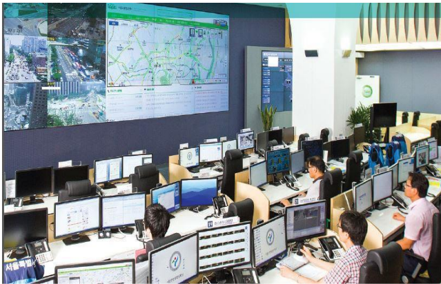
Fig. 5: Seoul TOPIS control room, interior view. Source: adopted from [31].
