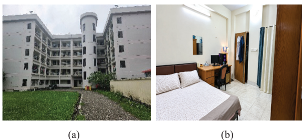
Fig. 1: (a) Exterior view of the case building; (b) Interior view of the corner room
