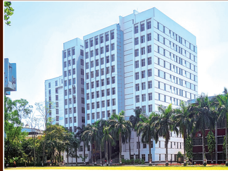
Shaheed Abu Sayed Administrative Building
